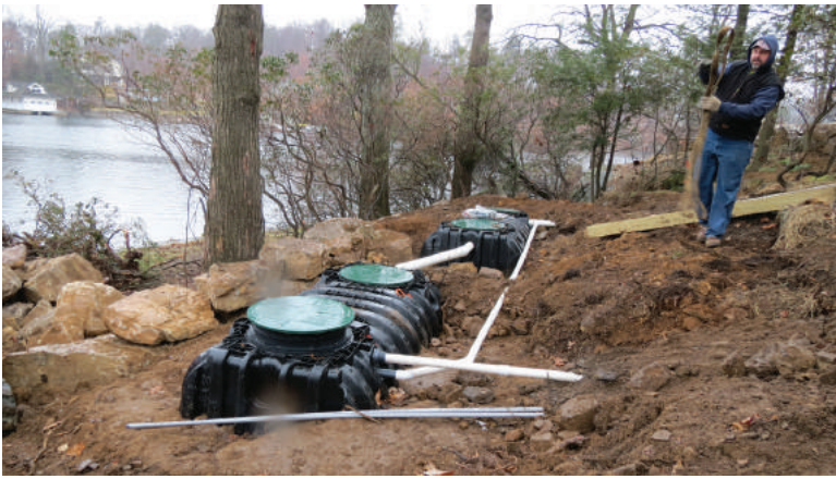
Bill Post of Septic Experts rolls up the rigging strap used to lift components and materials.
