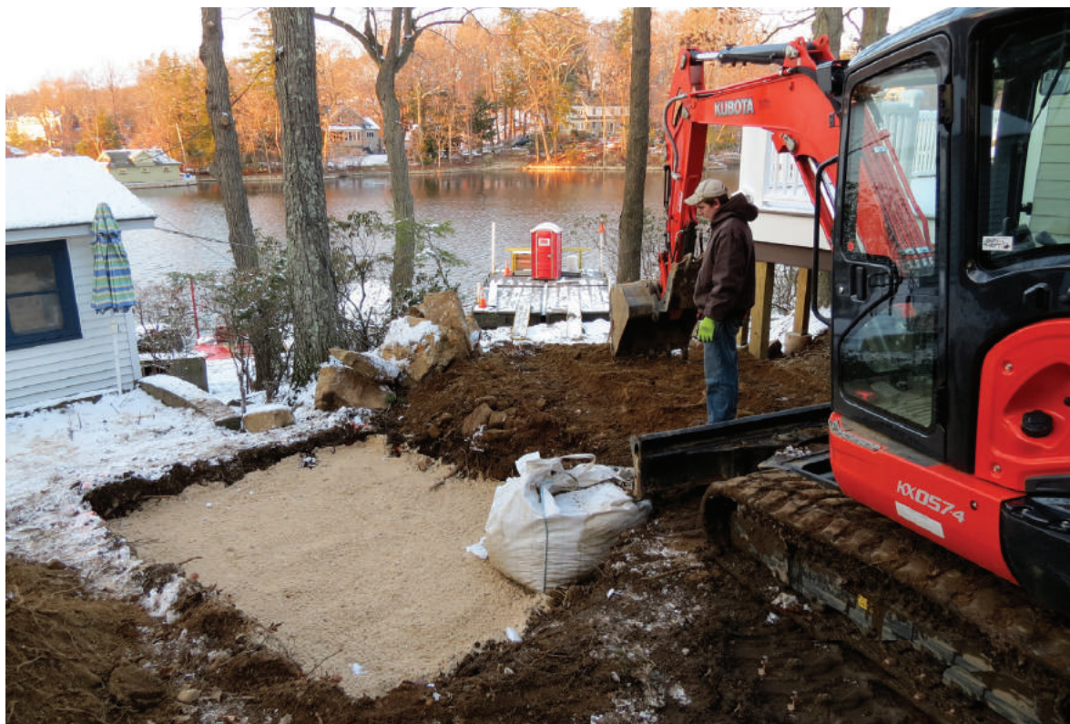
Avery Jinks of Septic Experts prepares to spread 3/4-inch crushed stone over the sand for the absorption bed. Some 20 feet below him is the barge with a portable sanitation unit.
