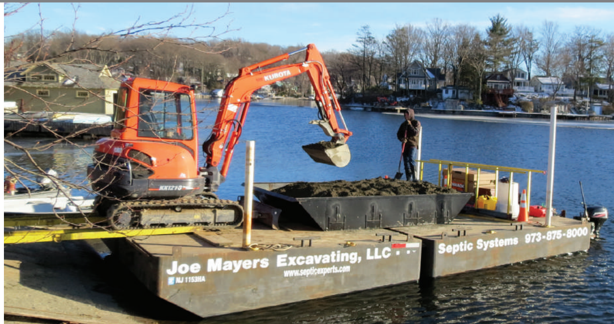
Using a Kubota 121 excavator, Bill Post of Septic Experts places screened fill in a 14- by 7- by 2-foot-high containment pan on a barge for transport to Raccoon Island. (Photos courtesy of Septic Experts)
