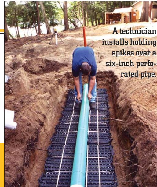
**A technician installs holding spikes over a six-inch perforated pipe.**
