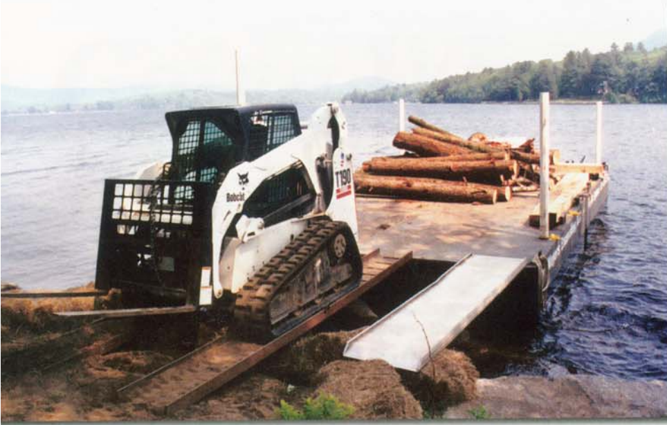
Loading logs from island onto the barge to bring back to mainland.
