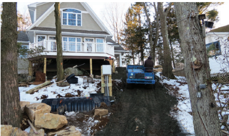
Avery Jinks of Septic Experts eases the IHI 1.3-cubic-yard IC30 crawler carrier up the steep slope past the septic tank and control panel to deliver another load of bank run.
