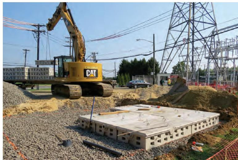
5.5-foot-deep drainfield. Dump trucks filled the hole with 4.5 feet of C-33 concrete sand and 12 inches of 1.5-inch crushed, washed stone, and hauled away spoil.
