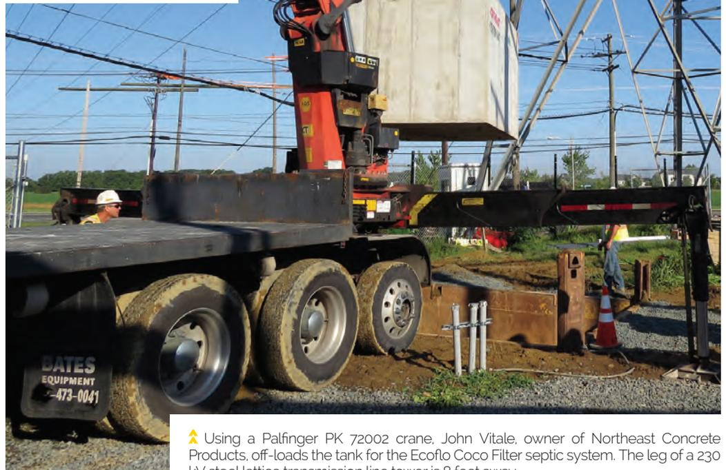
▲ Using a Palfinger PK 72002 crane, John Vitale, owner of Northeast Concrete Products, off-loads the tank for the Ecoflo Coco Filter septic system. The leg of a 230 kV steel lattice transmission line tower is 8 feet away.
